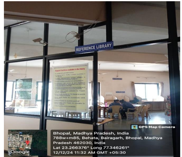
CCTV Camera installed at every corner of the college
